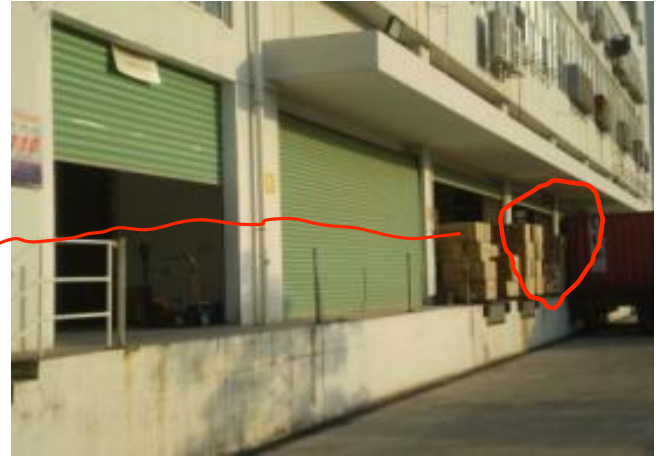
2. Container loading doors (external view)
