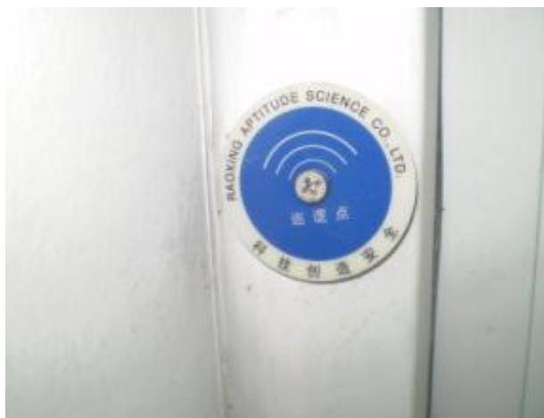
16. Security inspection magnetic point
